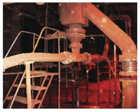
The solids-conveying venturi eductor has three ports: motive, suction, and discharge. The driving air from the main header travels through piping, enters through the motive port, travels through the motive connection, passes through the section chamber, carries the dust through the venturi and more piping, and discharges the dust into a silo.
