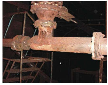
The venturi eductor has no moving parts, seals, or bearings, eliminating the chance for wear, increasing operator safety, and making it ideal for the company's application.
